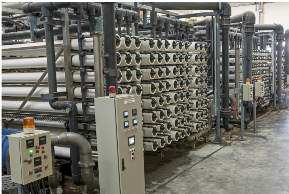
Figure F-2. Photograph of reverse osmosis system.
